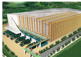
AS/RS Storage System China
