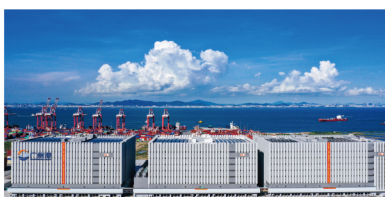
Cold Chain Logistics China
